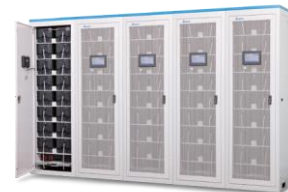
Cabinets in parallel
